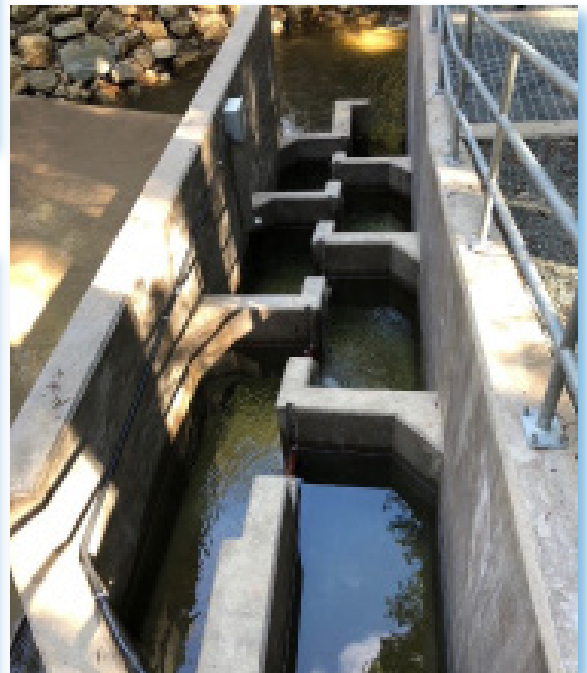
Inspecting the new fish ladder.
