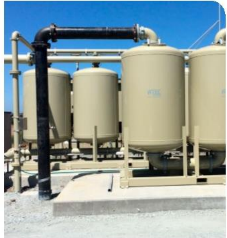
New vessels to increase the dosed chemical contact time
