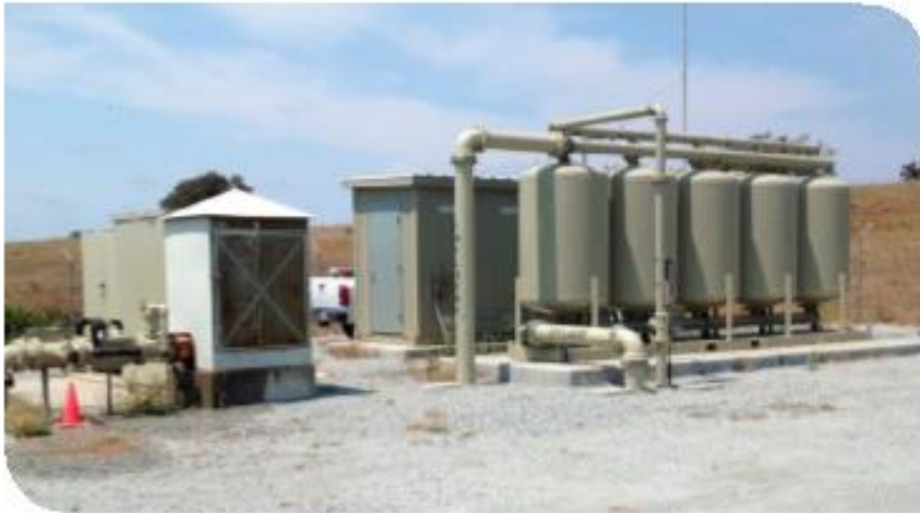
Existing Iron and Manganese Treatment Plant
