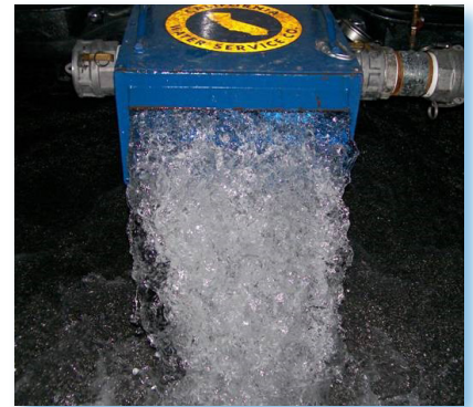
Cal Water Truck-mounted Diffuser with Dechlorination at the Beginning of a Flush and at the End
